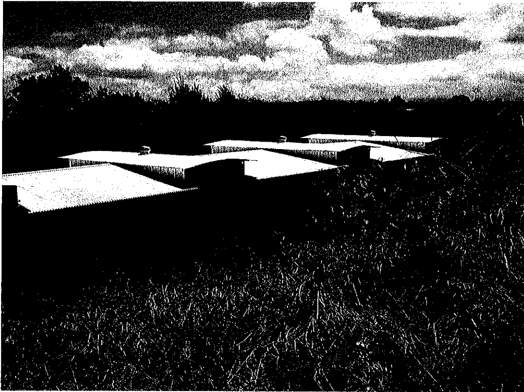
Fish hatchery operations container work space
